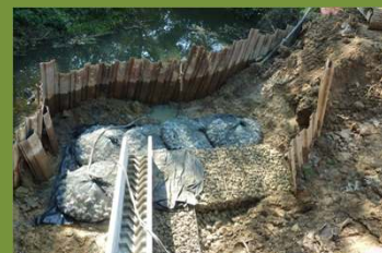
U.K. 2014 foot protection with gabion
