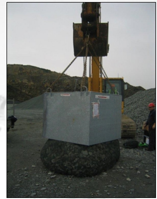
Lift production frame off the unit
