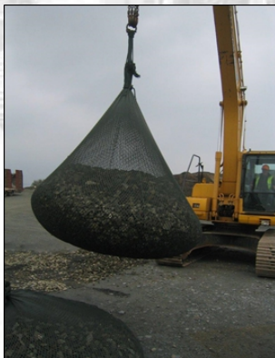
Lift using one point lifting ring to stock pile
