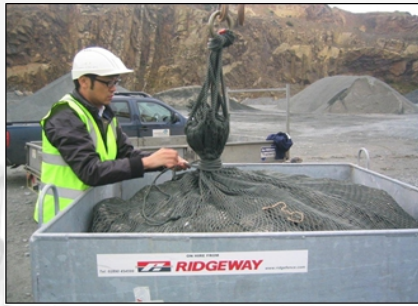
Attach forged steel ring and bind mouth
