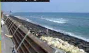
Works in progress
